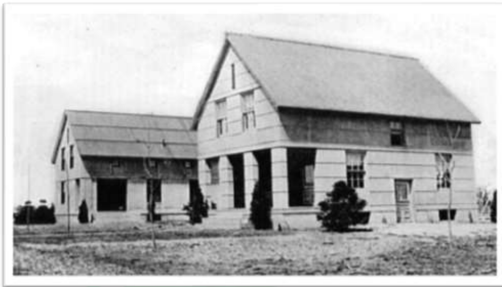
Fig. 1. One of G. Atterbury's experimental concrete houses in Sewaren, N.J. Photo by Standardized Housing Corporation / The Manufacture of Standardized Houses
